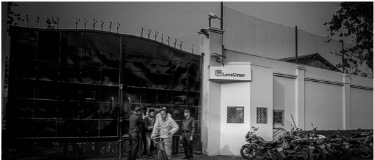
India Production Facility & Distribution Center for Australia, New Zealand, Asia Pacific & Africa. Moradabad, UP, India.
